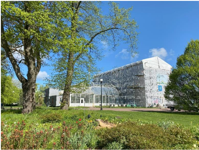
Figur 8: Palmhuset under renovering
